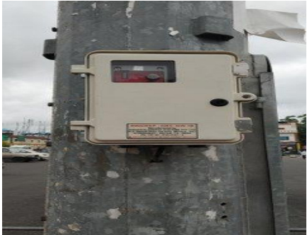
Provision of Timers for 30% & 70% High mast
